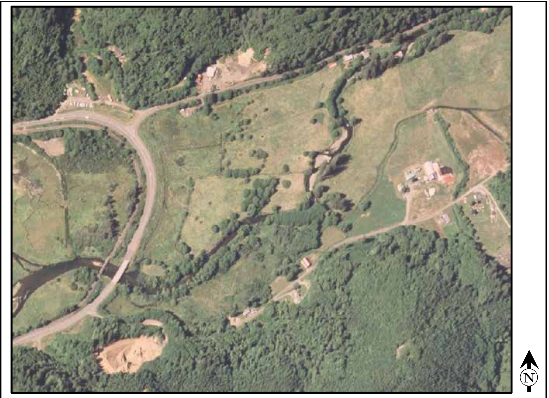
Figure 5. Recent, pre-project aerial photograph of Miami Wetlands Project site (ca. 2005). Note the two structures, the network of drainage ditches and the Hobson-Struby channel on the northern parcel. Also note the overhead utility corridor running southeast to northwest across the entire project area and the increase in riparian vegetation along the river as compared to Figure 3. Photo not-to-scale.
